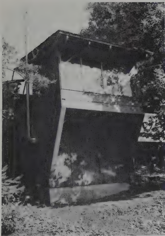
A compost privy built off the porch of a temporary dwelling. The permanent house was later built around this structure. One door leads to the in-use chamber, the other to the resting chamber. Rich humus taken from the privy is used to grow animal feed.
