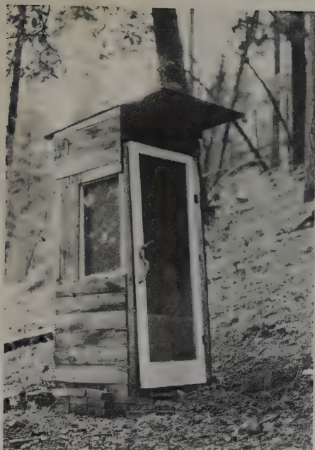
This pit privy has been serving a family of four whose code-approved septic system failed because of poor soil conditions.
