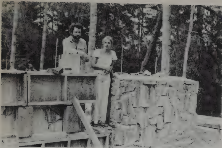
Mike and Sandy have spent three weeks of vacation plus every weekend for five months laying 90 tons of rock for the stem walls of their log garage/guest house. They plan to live in the guest house while taking five years to build their 2,750 sq. ft. log house.
