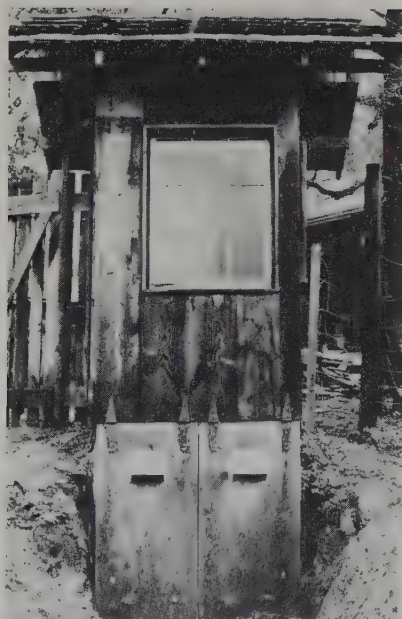
The prototype of the two-chamber D.S. Special composting privy, drawn above. State monitored tests of this system are in progress.
