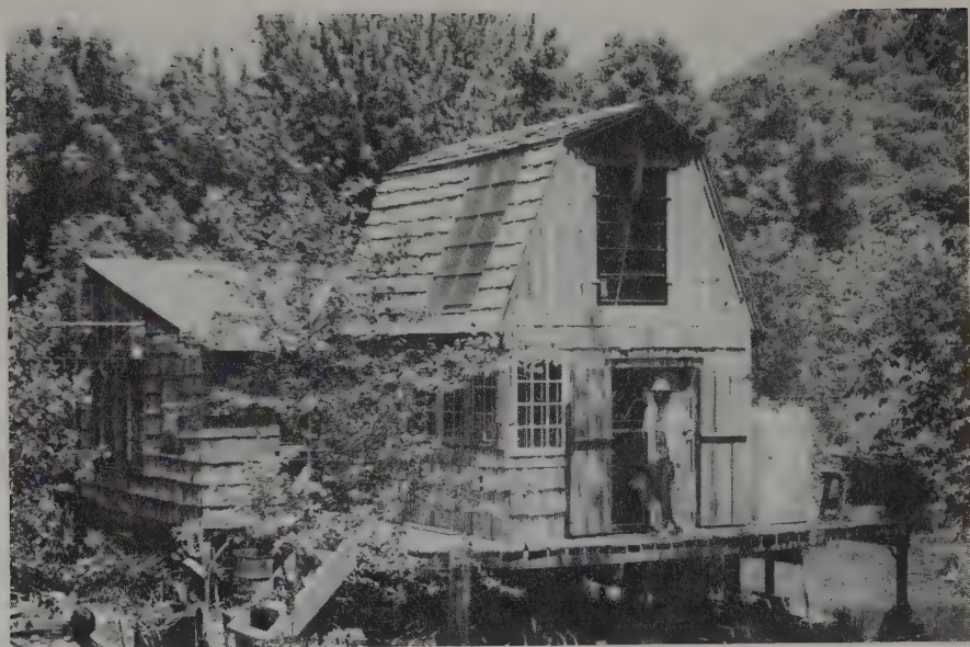
Dozens of 55 gallon drums and a system of vertical "gin poles" allow Leo Smith's house to rise and fall with the seasonal high water near the river.
