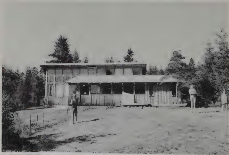
This owner-built house is well built and well designed in every respect except that the large bank of south-facing windows makes the space unbearably hot in summer. This mistake was made because the inexperienced owner-builder designed his house in the winter.
