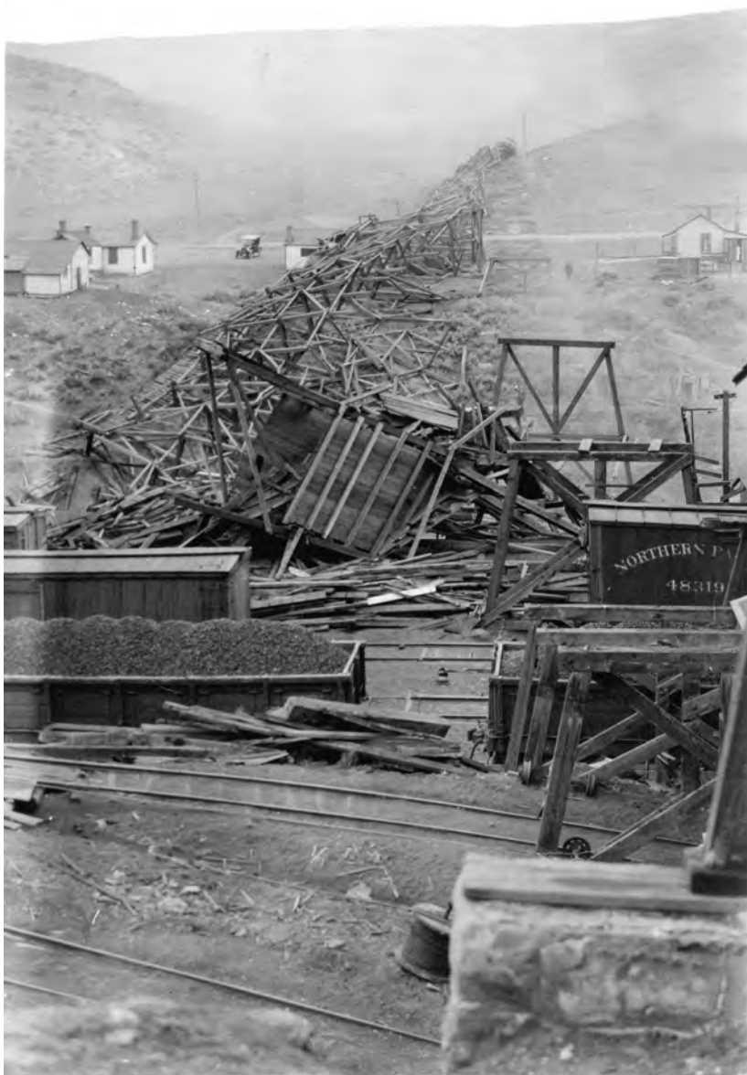
A windstorm in October 1920 destroyed the Bear Creek Coal Company's trestle that spanned the valley and allowed access to mine workings on the south side. This disastrous event led to the company's financial collapse a year later. (CCHS&M-Kidwell Collection).
