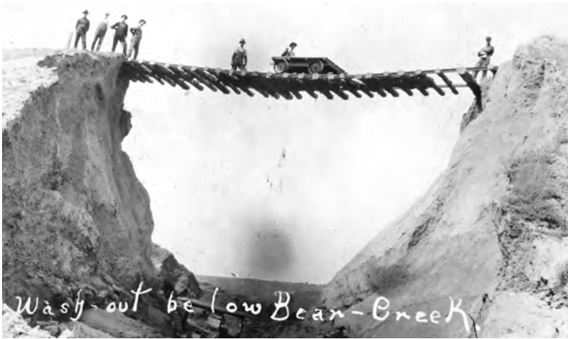
During its early years, the MW&S was plagued by numerous washouts like this one that occurred just east of Bearcreek near Mile Post 19 on September 4, 1912. (General Photograph Collection, Railroad Museum of Pennsylvania, PHMC).
