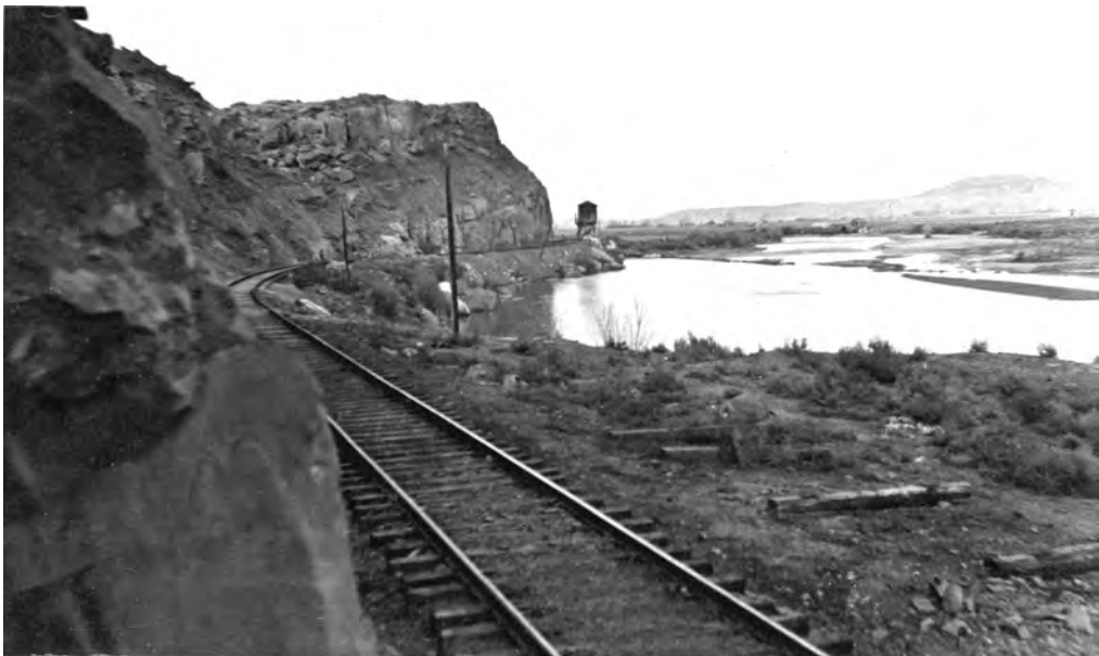
In this view looking north along the Clarks Fork River about one and a half miles from Belfry, the railroad's lightly ballasted but otherwise well-maintained roadbed can be seen along with the water tank that used a steam jet to draw water from the river. This may have been the area where locomotive Number 6 took its unfortunate plunge during July 1919. (General Photograph Collection, Railroad Museum of Pennsylvania, PHMC).
