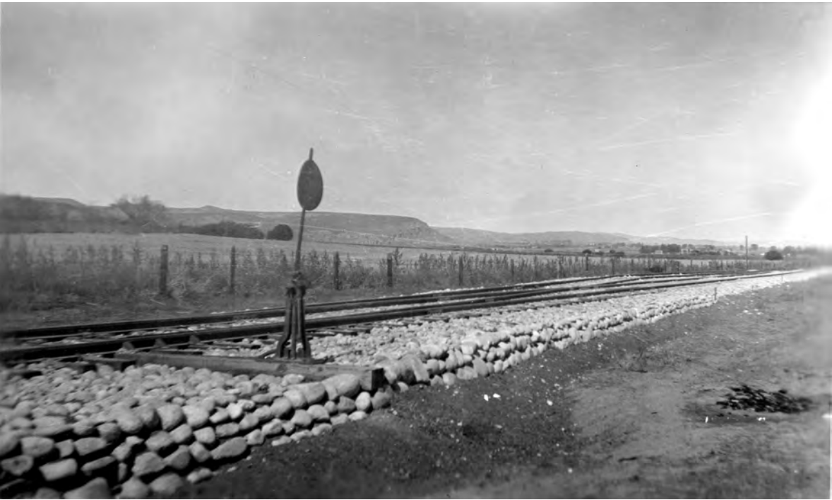
Edward Bunney's improvements to the MW&S included the addition of rock ballast. This view taken at the south end of the Belfry yard in September 1929 shows a section of line ballasted with neatly manicured river rock. River rock appears to have been widely used by the MW&S as anomalous rounded cobbles can still be found along many parts of the old roadbed. (General Photograph Collection, Railroad Museum of Pennsylvania, PHMC).
