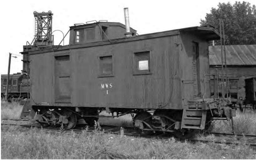
Yellowstone Park Railroad caboose Number 1 was a short, home-built, side-door design completed in early March 1907. Still in service forty years later, it is seen here in the Belfry yard. (Courtesy of California State Railroad Library & Archives).
