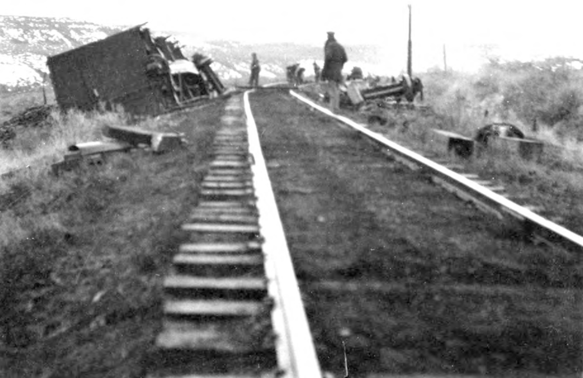
This undated photo shows an all-too-common occurrence during the early years of operation. A runaway boxcar has left the rails on a curve somewhere in the Bear Creek Valley. Although the ties appear to be in good shape, the railroad's "mud ballast" is clearly evident. (CCHS&M-Kidwell Collection).
