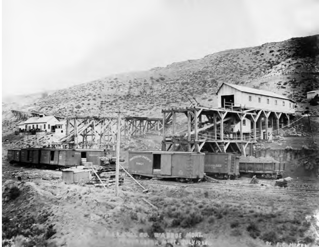
Montana Coal & Iron's Foster Gulch mine began full-scale operation in 1917. This photo, taken in 1920, shows the three tracks beneath the tippel used for loading different sizes of coal. The track nearest the hillside was used for slack. Cars on the other two tracks would have received nut or lump coal. To the left is the uncovered tippel used by the Eagle Coal Company, which hauled coal from its mine portal farther up the gulch to the tippel via an electric tramway. A small section of the tramway is visible behind the building on the far left. (Lot 026 B6F3.12, NP rail cars in front of Foster Creek Mine, Montana Historical Society Photograph Archives).
