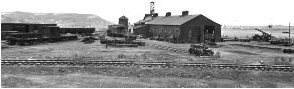
This view of the engine house and yard facilities in Belfry is to the north. The water tank and the top of the coaling tower are visible just beyond the engine house. The tracks in the foreground connect the mainline to the Bear Creek branch and form the wye used for turning locomotives. (General Photograph Collection, Railroad Museum of Pennsylvania, PHMC).
