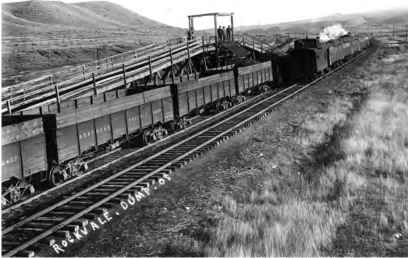
This sugar beet dump near Rockvale on the NP Rocky Fork Branch is similar to beet dumps on the MW&S located on Golden Flat and just north of Belfry. (L. G. Webber photo, Joliet Public Library).
