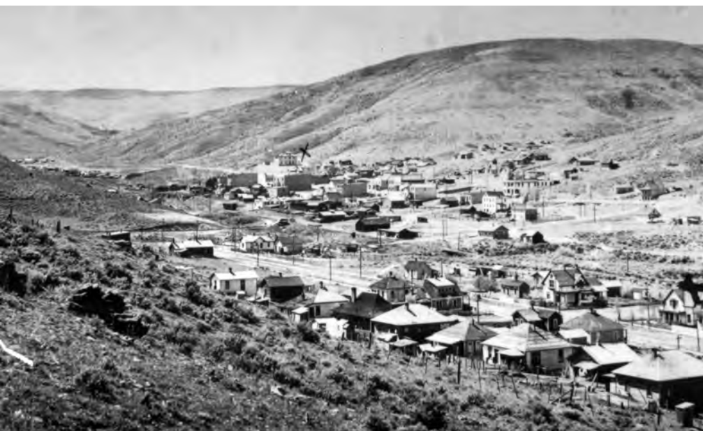
This northwesterly view of Bearcreek taken in 1918 shows the recently completed Foster Gulch wye in the bottom of the valley, one leg of which departs the mainline to the right of the short trestle visible in the lower right. The other half of the wye can be seen cutting across the hillside in the center left. The MW&S depot is located trackside just to the left of the trestle at the corner of Fourth Street and First Avenue South. Virtue Gulch is visible in the upper left. (CCHS&M).
