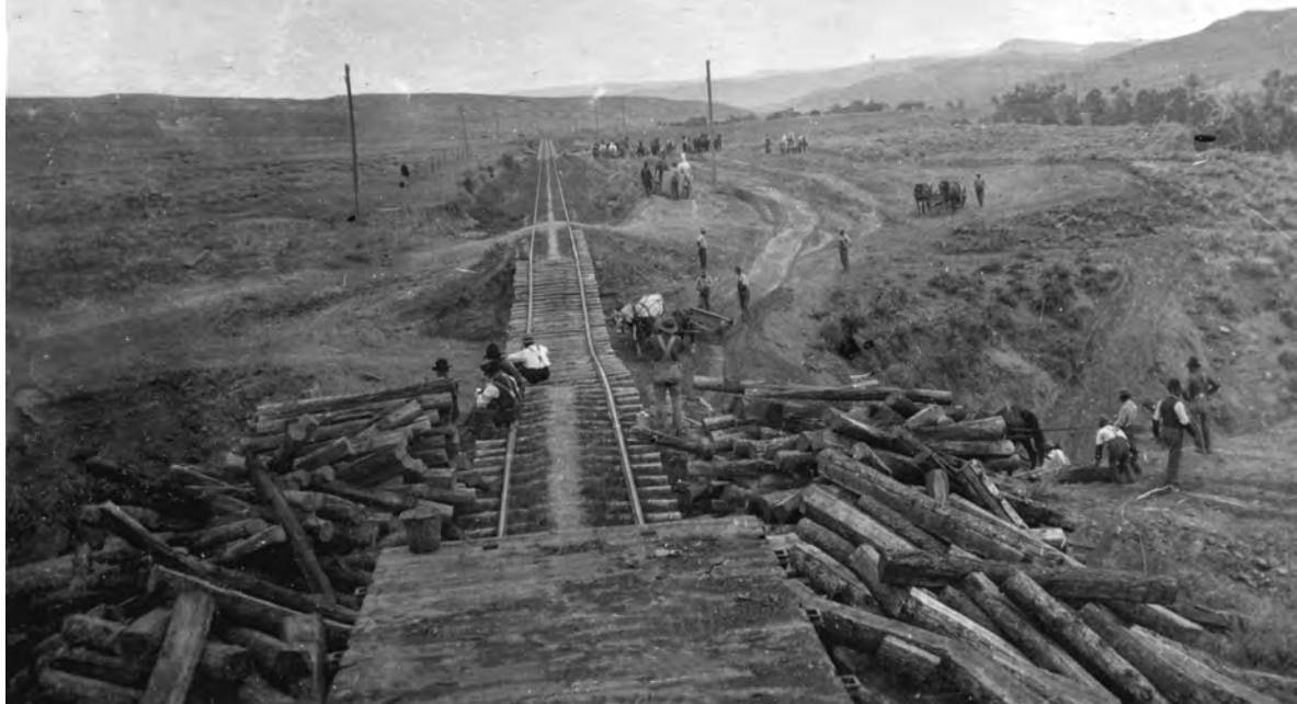
At least ten horse teams and more than a dozen men are hard at work repairing damage to the line about three and a half miles west of Belfry. This undated photo looking east down the Bear Creek valley illustrates one of the railroad's recurring problems: washouts that were a direct result of its narrow, poorly drained, unballasted roadbed. (CCHS&M-Kidwell Collection).
