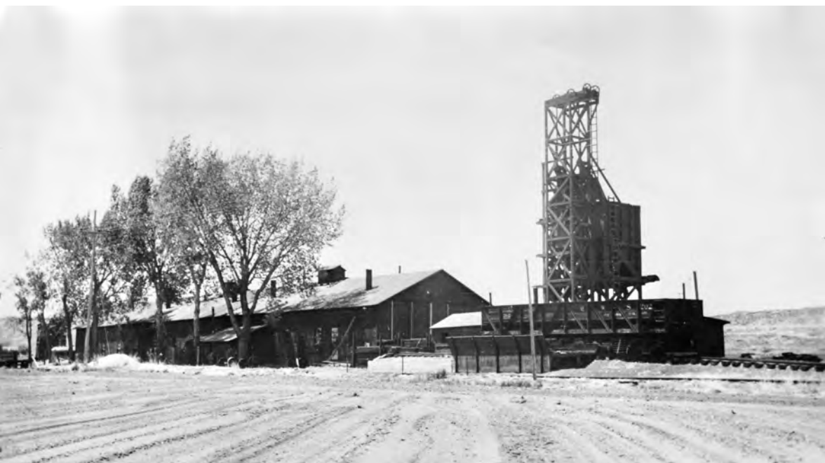
This 1954 view of the north end of the engine house reveals the railroad's unique coaling tower with its numerous external cables and sheaves. A drop-bottom gondola is visible on the unloading ramp at the base of the structure. (PAC 97-93.14416 MWS Shop-Coal Dock Belfry 5/1954. TTT, Montana Historical Society Photograph Archives).
