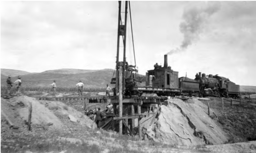
This photo shows MW&S locomotive Number 5 working with an NP pile driver to replace a damaged trestle. Although the location of this photo is uncertain, this may be the trestle that was damaged by fire in December 1919, or it may simply have been the victim of a cloudburst and flash flood. (CCHS&M-Kidwell Collection).
