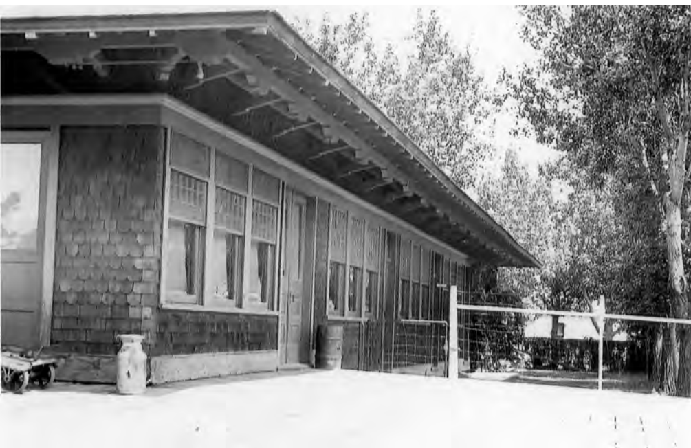
The architectural details of the Belfry Depot are evident in this view from 1931, which include three types of decorative shingles on the walls, scrolled rafters, and beveled soffits. (CCHS&M).
