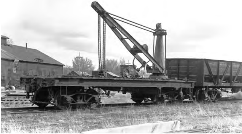
This MW&S "armstrong" derrick car was built for the Yellowstone Park Railroad in 1906. The frequency of derailments during the early years of operation must have kept this piece of equipment busy. It is seen here in Belfry during May 1955 just prior to being scrapped. (PAC 97-93.12758, MWS Derrick car, Montana Historical Society Photograph Archives).
