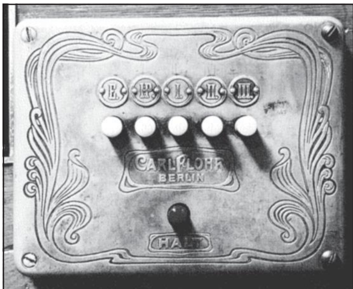
An example of the early push-button system. From Kerstin Englert and Alfred Englert, Lifts in Berlin (Berlin: Jovis, 1998).
