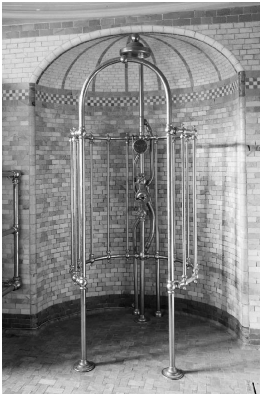
Fig. 5.2. A shower at Ardkinglas, Argyll, United Kingdom; fitted in 1906, it features wave and spray controls. The house was completed in 1907 for the armaments dealer Sir Andrew Noble to designs by Sir Robert Lorimer. The house remains in the family. Published in Country Life , 29 September 2010.
