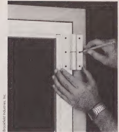
12-6 Use the hinge as a template.
