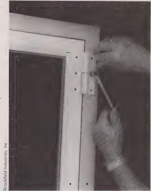
12-9 Expand the fasteners.
