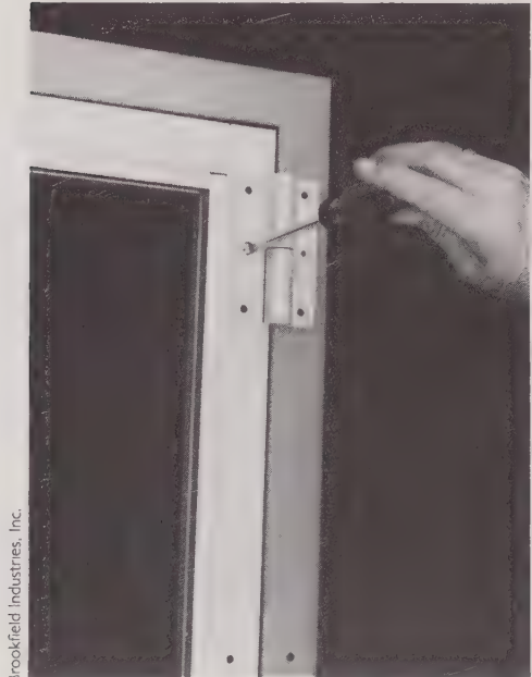
12-10 Install steel screws.
