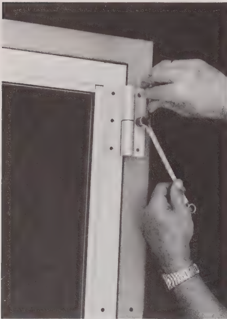
12-8 Insert a blind threaded fastener.
