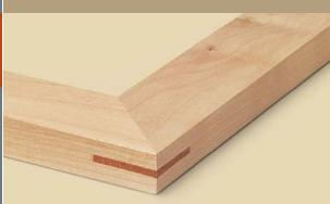
Splines are cut prior to the joint being glued. They strengthen the joint by providing a face-grain glue surface.
