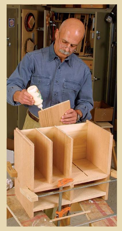
ASSEMBLE THE PIECE. Begin by gluing the sides to the two shelves. Apply some glue to the grooves and slide in the drawer divider from the front. Then slide in the back slats and glue in the partitions. The last piece of the case to be attached is the top. Working on a pair of sawhorses gives you more options for clamping positions.
