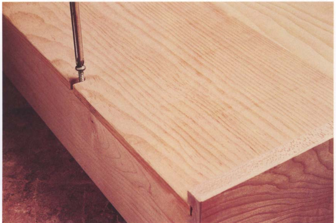
Photo L: When installing a solid-wood drawer bottom, allow for wood movement by cutting slots for the screws.
