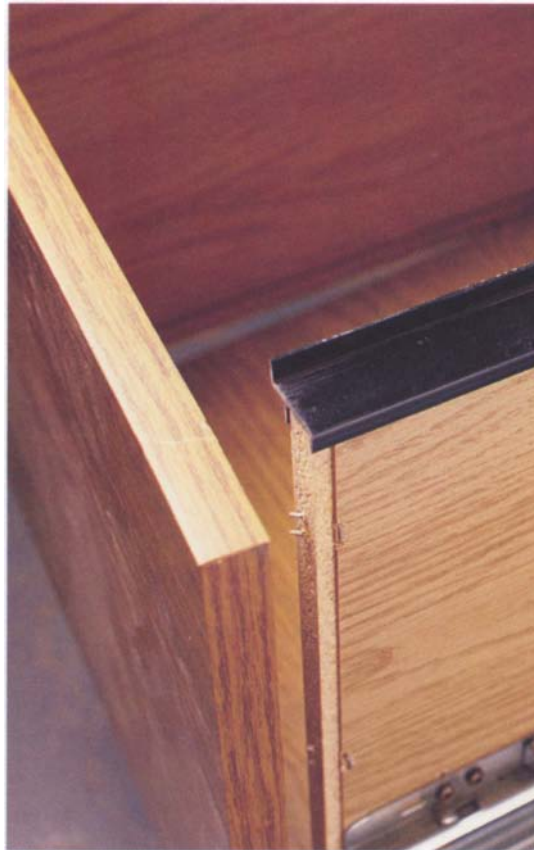
Particleboard, often used in low-grade commercial furniture, doesn't hold fasteners well, particularly in end-grain applications like this drawer joint.
