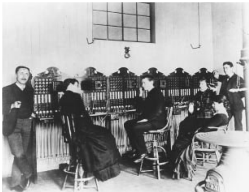
Figure 3.6 Telephone Operators. This is a very early photograph of telephone operators, dating from 1883. Taken in Boston, it shows men and women working together at a switchboard. The operators connected calls by attaching the caller's line to the appropriate slot in the plugboard that is mounted against the wall. Within a few years, this job would be reserved for women, the famous "hello girls." Automatic telephone switching became commonplace in the 1920s, after having been long resisted by AT&T. AT&T executives worried that customers would resent having to dial calls themselves; they also sought to protect the firm's enormous investment in manual switching equipment. Courtesy of AT&T Archives.
