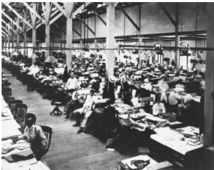
Figure 4.3 Census-Taking as Big Business. In this 1910 photograph we see the main working room at the U.S. Bureau of the Census, loaded with Powers's Automatic Electric Card Punch equipment—the arch-rival of the Hollerith Tabulating Machine Company—along with some of Hollerith's smaller devices, such as the Pantograph Punch on the table in the lower foreground. What is important to note in this picture is the extent of the commitment to information technology that a government agency had to make in order to do one task—in this case, census taking—while other agencies were also embracing the new technology. Courtesy of the National Archives.
