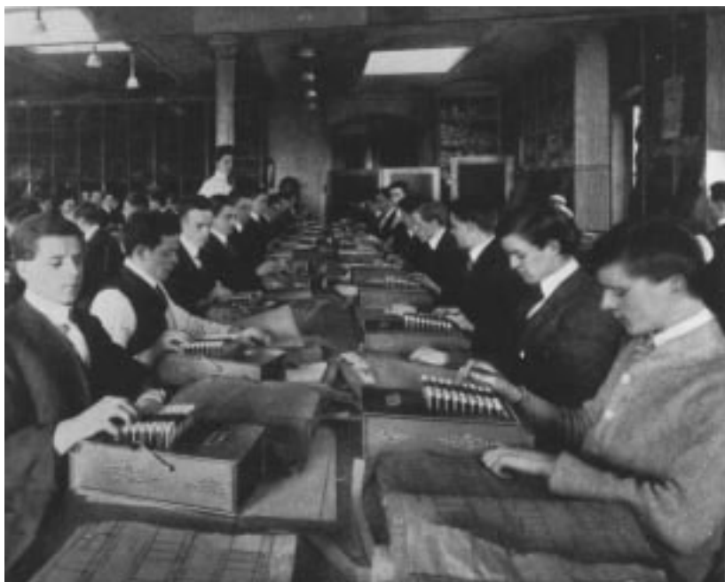
Figure 4.2 Calculating Accountants. Nothing so profoundly changed the job functions of an accountant, or did more to expand the types of accounting that could be developed and applied, than the humble adding machine. In this picture, the Comptometer, the most popular calculator among accountants of the period 1900–1930, is used by members of the audit team at the Pennsylvania Railroad. The Comptometer was particularly useful in conducting a variety of basic mathematical functions in large enterprises. Manufactured by the Felt & Tarrant Company, it was the most important competitor to another great American firm, the Burroughs Adding Machine Company. From the private collection of James W. Cortada.
