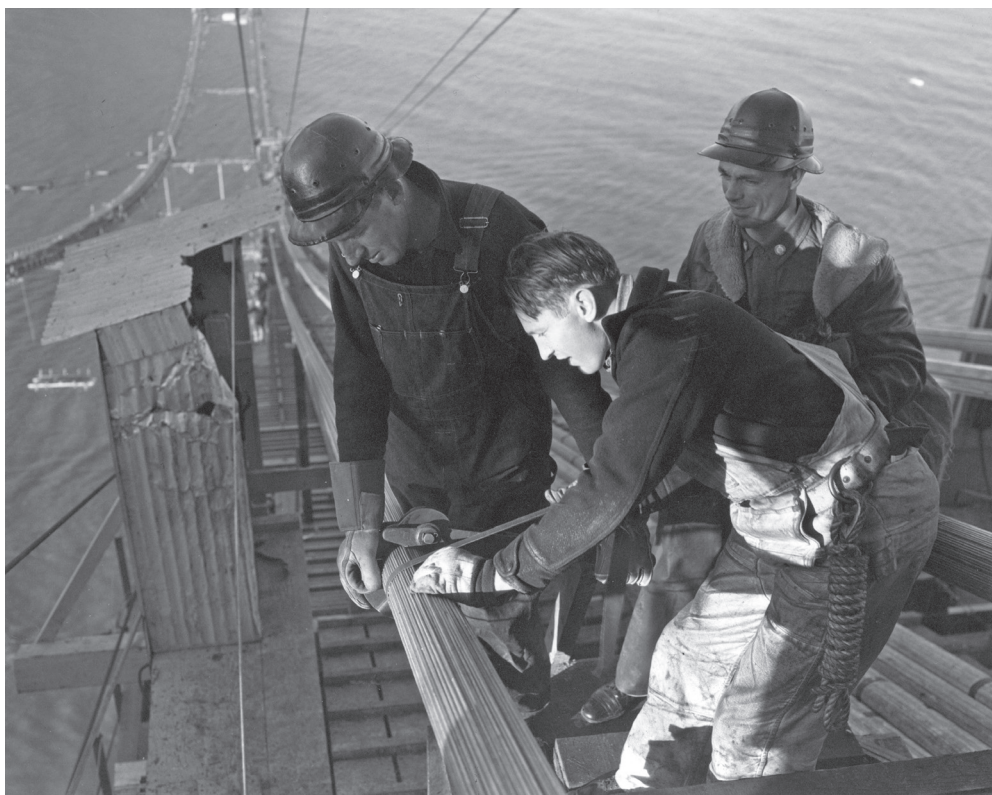
Fred Dummatzen ( left ) and coworkers banding cable strands on the bridge, 1936. Martin Adams sadly recalled the terrible accident on February 17, 1937, that killed Dummatzen and nine other men. Photo by Charles Hiller. Courtesy of Labor Archives and Research Center, San Francisco State University. Copyright Golden Gate Bridge, Highway, and Transportation District.
