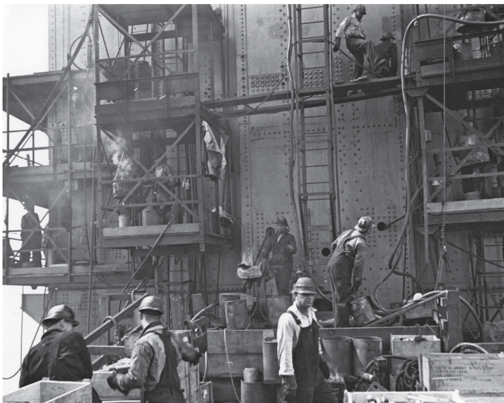
Heaters and riveters at work on the Golden Gate Bridge. The intense construction activity awed Fred Divita when he began his first day on the job in 1934. Photo by George Douglass. Courtesy of Labor Archives and Research Center, San Francisco State University. Copyright Golden Gate Bridge, Highway, and Transportation District.
