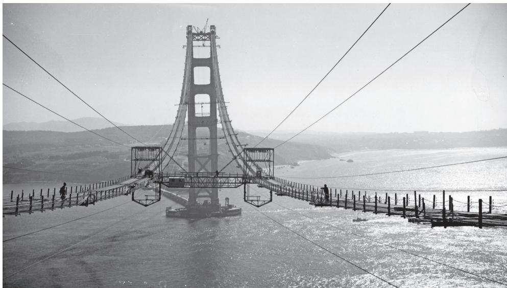
Catwalks under construction, 1935. One windy day Fred Brusati feared that the catwalk he was on might flip over, but he was wearing a safety belt and thought he would survive. Photo by Ted Huggins. Courtesy of California Historical Society, Huggins Collection, CHS.Huggins.033.
